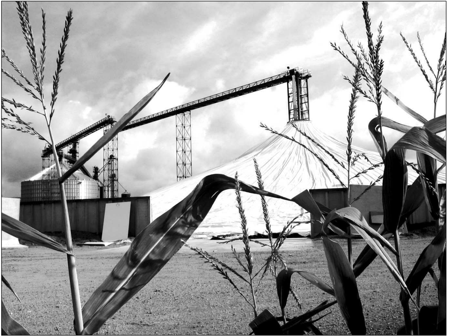
The tasselled corn adjacent to the expanded bunker at Minnesota Falls frames the tarped grain pile already holding corn awaiting delivery to Granite Falls Energy. The bunker will hold 3.5 million bushels of corn that will flow into the facility under the winched tarp.
